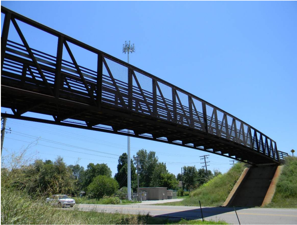
3.2 Example of a pre-engineered pedestrian truss bridge over IL 162 near Troy
