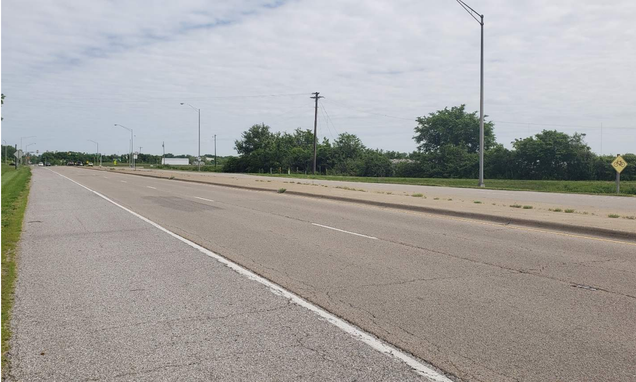
Photo 1: IL 111 looking North towards Schoolhouse Trail
