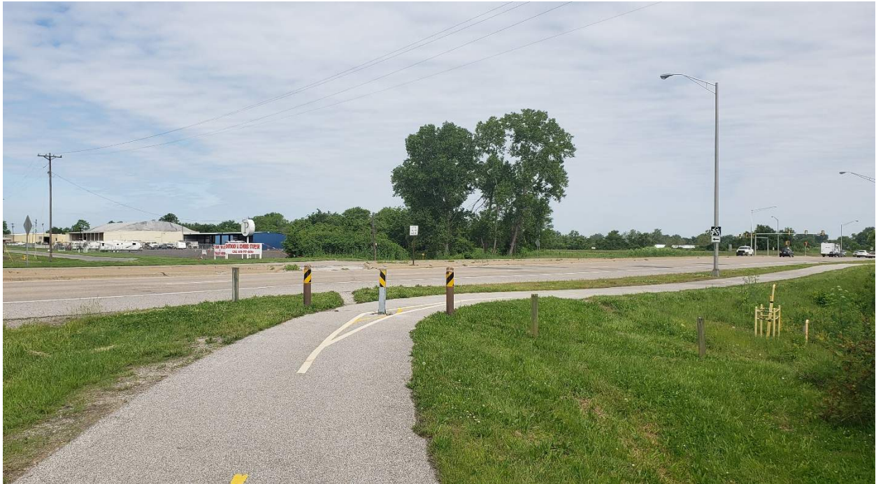
Photo 3: Schoolhouse Trail (East) looking West towards IL 111
