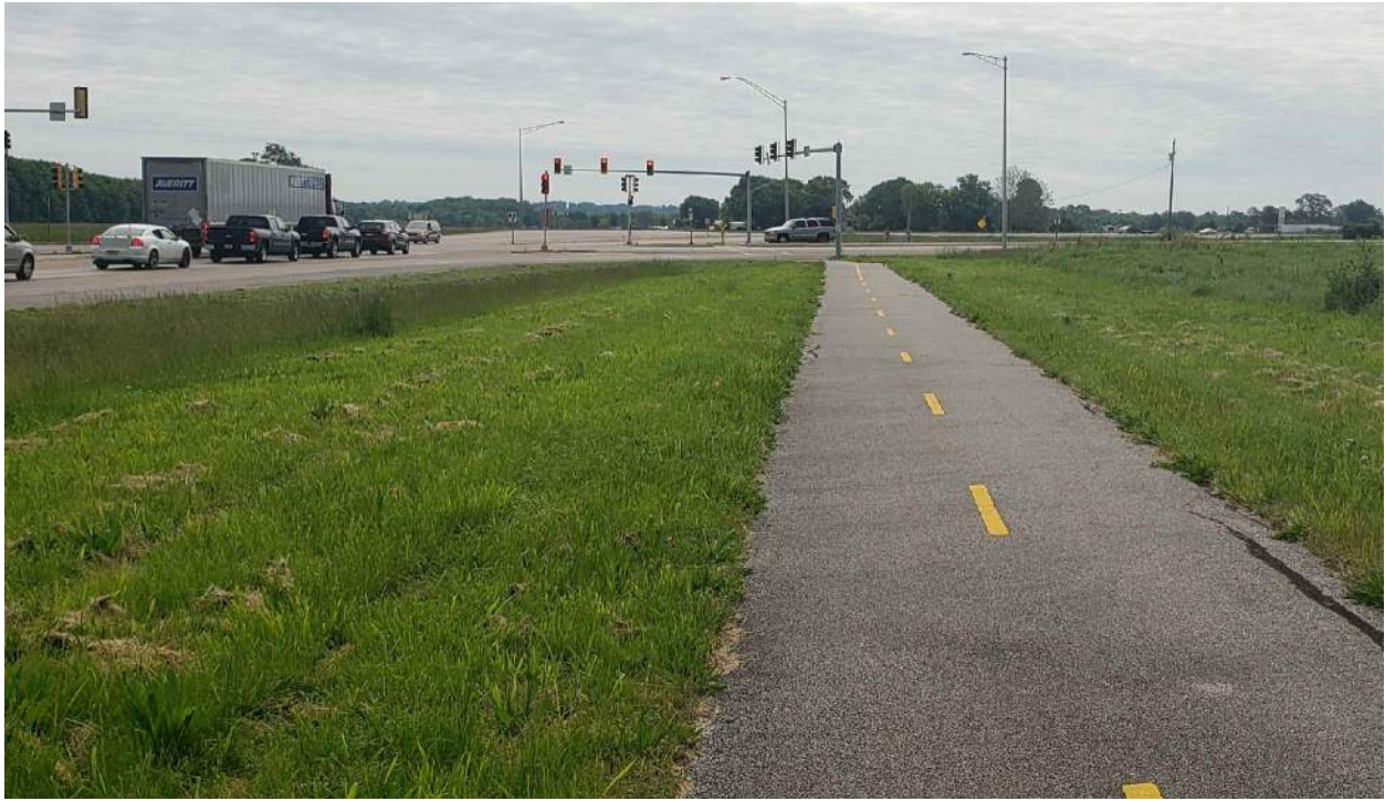
Figure 9: Looking East towards IL-111 / Horseshoe Lake Road
