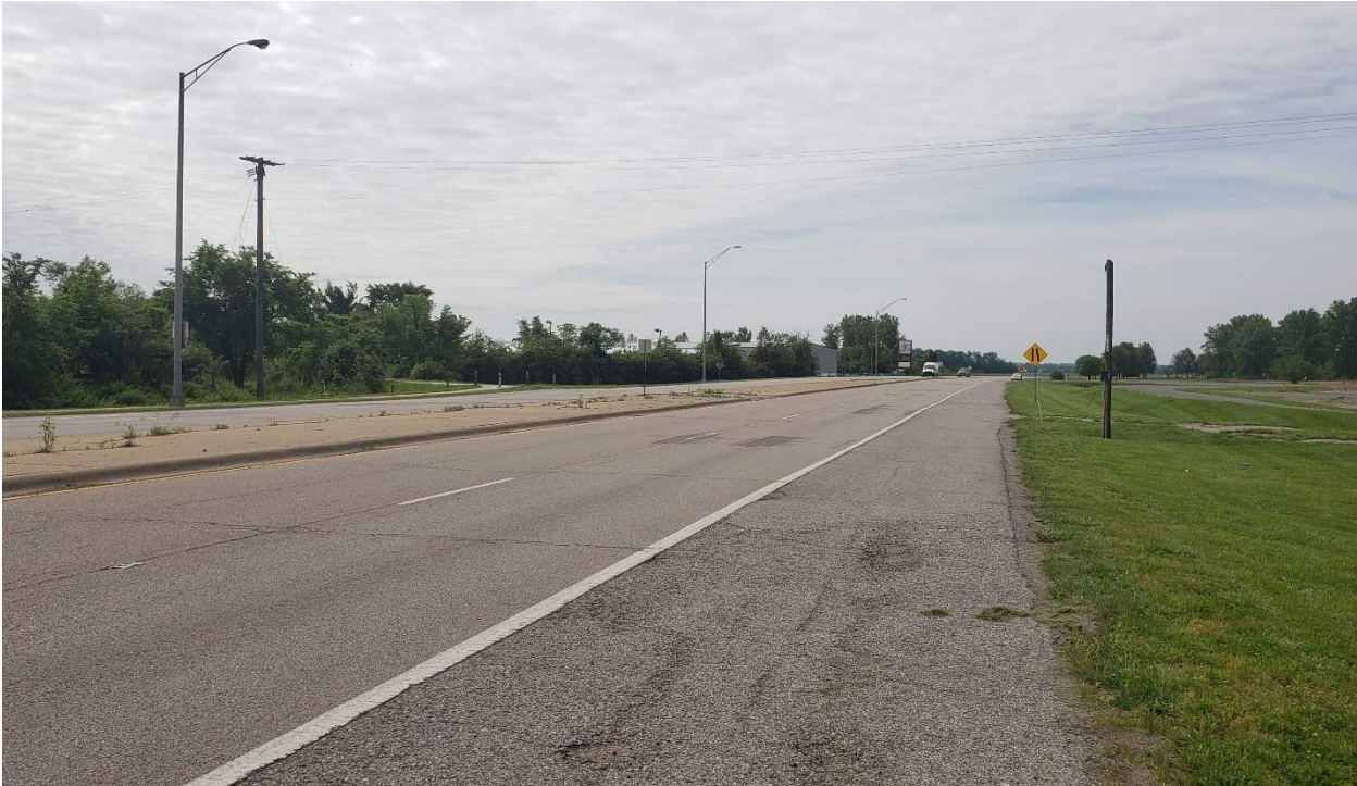
Photo 2: IL 111 looking South towards Schoolhouse Trail
