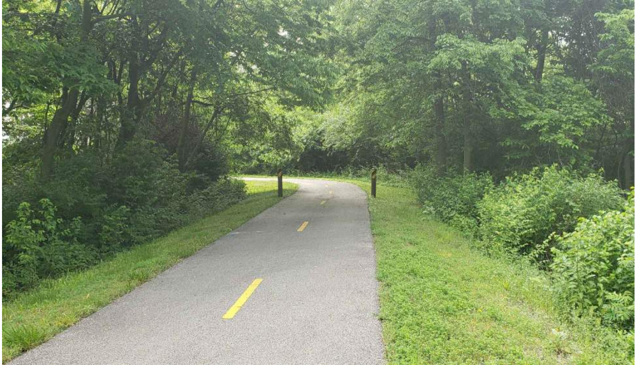
Figure 3: Schoolhouse Trail (West) looking East towards IL-111
