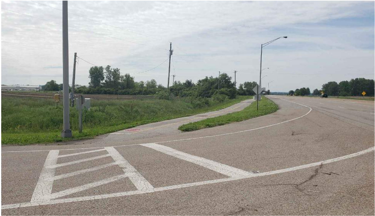
Figure 7: IL-111 / Horseshoe Lake Road looking South along Schoolhouse Trail
